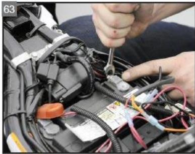
63 Install and tighten the negative battery cable.
