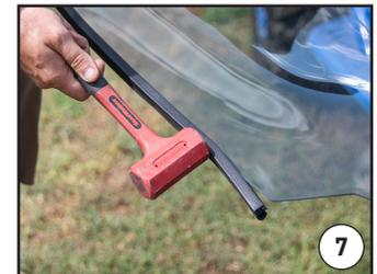
5. Place black plastic washers on both studs. 6. A single piece of trim has been supplied to cover the bottom of the Flare™ Windshield. 7. With the bulb facing the back side of the windshield, install trim on the lower lip. A rubber mallet may be needed to fully seat the trim (**BE GENTLE**).
