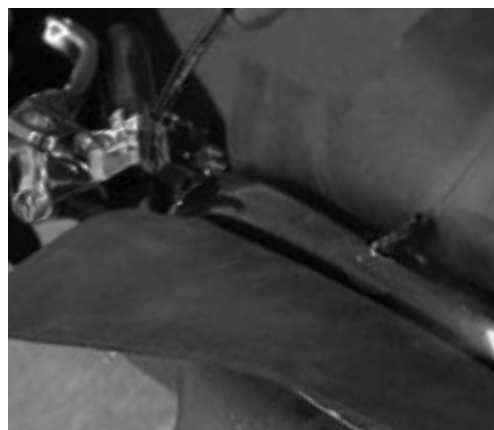
PHOTO 11 (BARS SHOWN FROM BOTTOM)
